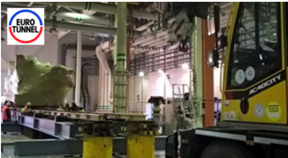
Transporting and rigging of the CenTraVac™ Chillers to the jobsite of Eurotunnel.
